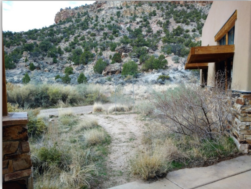
View at the rear of the smaller building which can open to a visitor trail.
